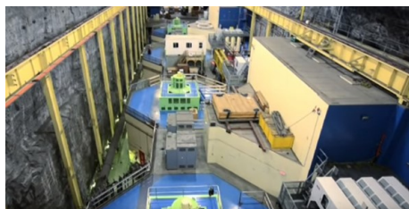
Northfield Mountain storage facility | Northfield Mountain
