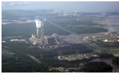
Brandon Shores power plant
