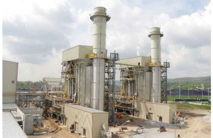
Cane Run Unit 7, a fast-start 640-MW combined cycle plant, went into service for Louisville Gas and Electric and Kentucky Utilities in 2015. | © RTO Insider
